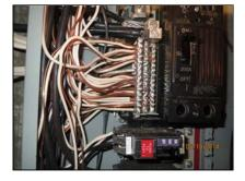
(3) The main service panel and/or its components requires immediate action to minimize the possibility of electrical shock. There are missing knock-outs in the panel enclosure. Properly cap/seal openings.
