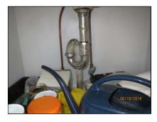
(3) The bathroom sink drain popup assembly is not properly operable. Repair as necessary.
