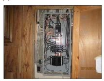
(2) There appears to be a wiring problem in the service panel that calls for immediate action. There are ground and neutral conductors or just neutral conductors in the main service panel that improperly share the same attachment screw. Properly separate the ground and neutral conductors with each conductor attached by independent screws.
