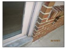
(2) The main entry door is deteriorated. The frame/door or threshold is seriously deteriorated due to prolonged exposure and inadequate maintenance. Have a qualified contractor properly repair/rebuild/replace as necessary..
